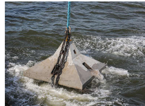
Bio-facilitating anchor during installation.
