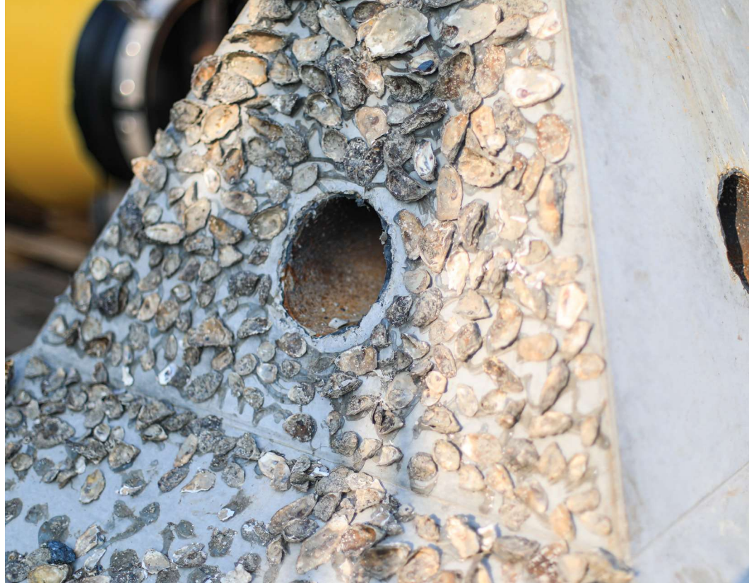
Bio-facilitating anchor with oyster shells as substrate and holes to serve as shelter for organisms.
